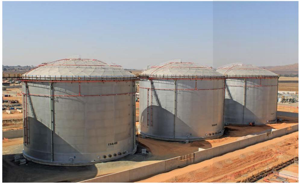
ALUMINUM DOME AND INTERNAL FLOATING ROOF
